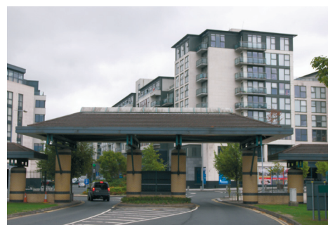
EXISTING 9-10 STOREY BUILDINGS BESIDE TALLAGHT HOSPITAL ENTRANCE & HELIPAD
